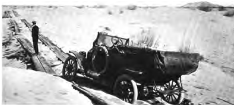
Before the era of the State Highway parallel planks served for a road.
